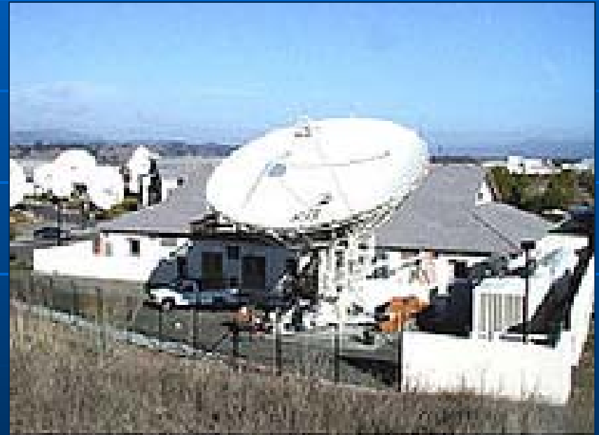
GPS Facility in Napa, California
