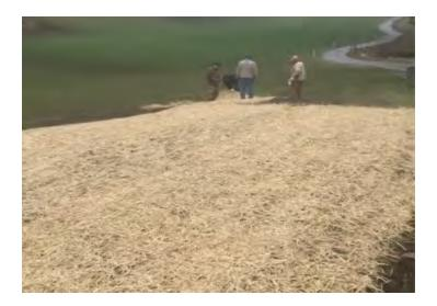
Figure 2. Care should be taken during turfgrass establishment to minimize erosion potential. Photo Credit: John Jacob.
