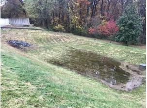
Figure 11. Retention areas allow stormwater to infiltrate into the ground. Photo Credit: John Jacob.
