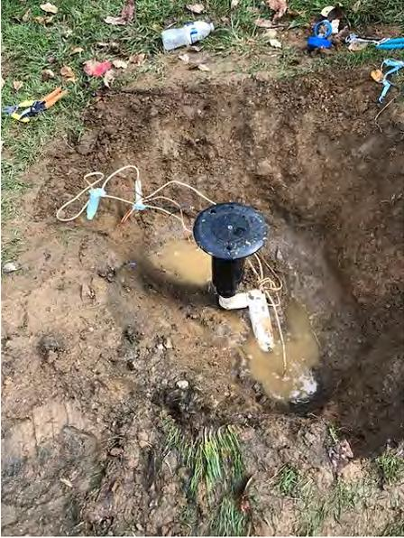
Figure 8. Irrigation system maintenance and repair conserves water and protects turfgrass. Photo Credit: John Jacob.
