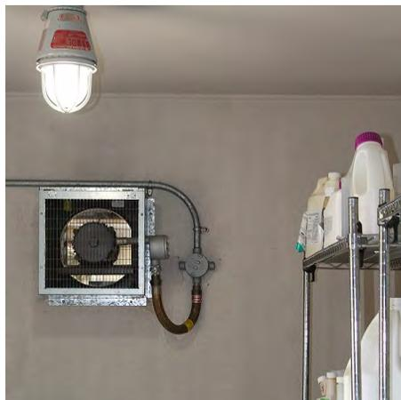
Figure 20. Pesticide storage areas must be adequately ventilated. Photo Credit: Erik Ervin.
