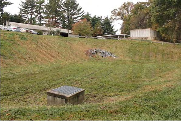
Figure 12. The retention area is usually empty of water. Photo Credit: Erik Ervin.
