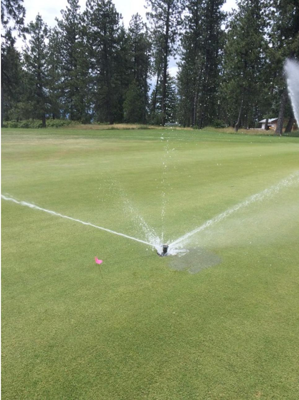
*Figure 5. Regular auditing of the irrigation system should be performed to check actual water delivery and nozzle efficiency.*
