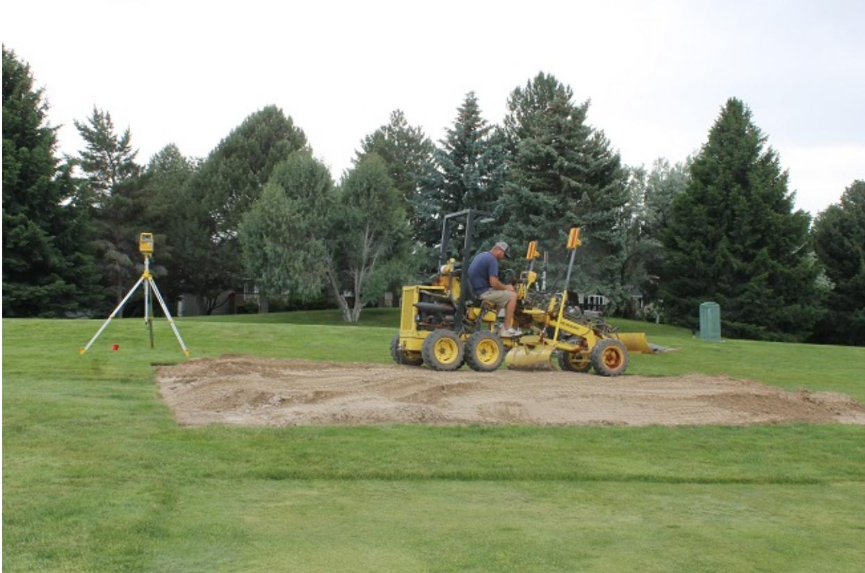
*Figure 3. Grading the surface prior to planting.*
