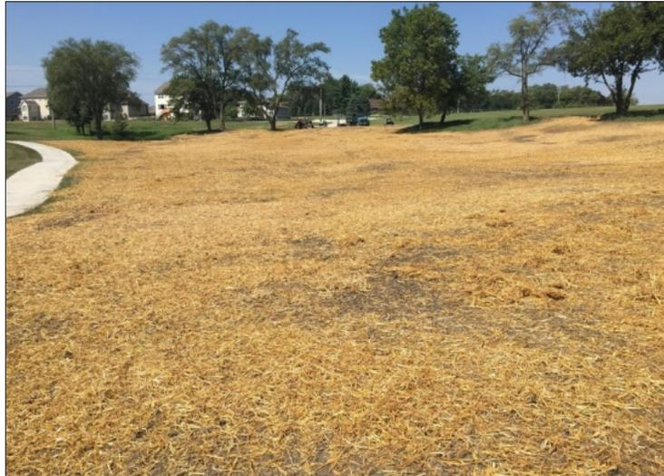
*Figure 2. Straw is used to protect soil and seed from water erosion.
