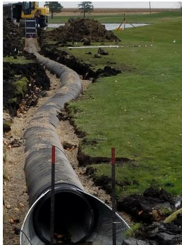
*Figure 17. Drainage pipe installation.
