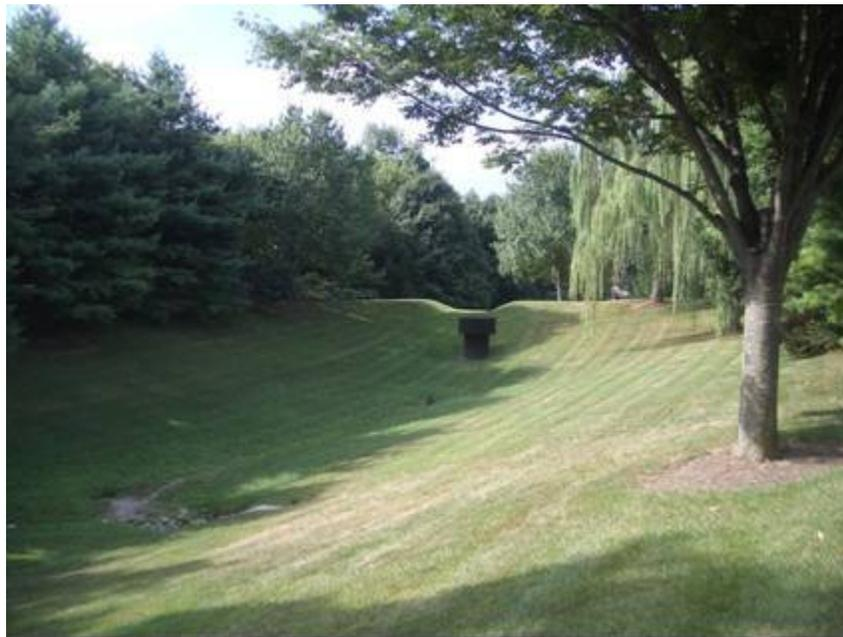
*Figure 8. Use dry detention basins/catchments to buffer flooding and excessive runoff that may contain sediment. Photo credit: Kraig Binder.*
