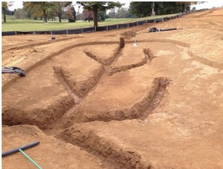
*Figure 2. When constructing drainage systems, pay close attention to engineering details such as subsoil preparation, the placement of gravel, slopes, and backfilling.
