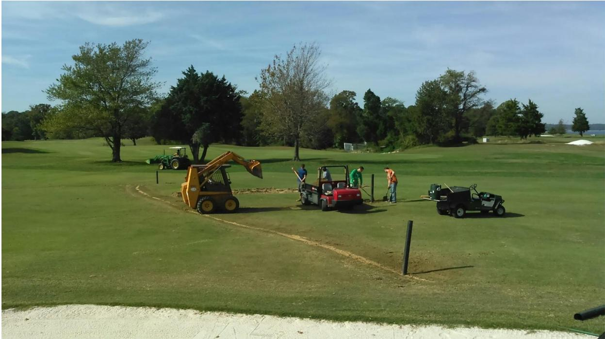
*Figure 7. Drainage project on #18 fairway at Cedar Point Golf Course. Water is carried back and empties into an irrigation pond providing up to 1 million gallons of recovered rainwater each year. Photo credit: David Burkhart.*
