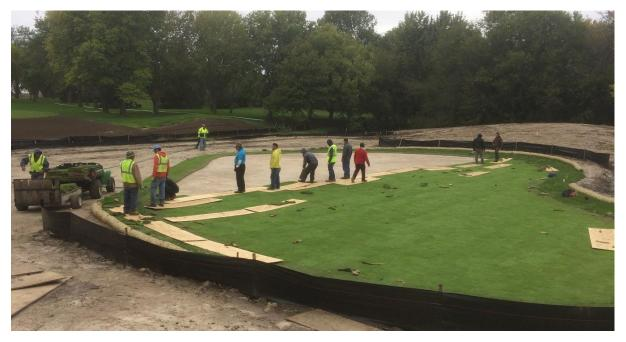
Figure 2. Erosion and sediment control during construction helps to protect water quality from runoff during construction at Oak Hills Country Club. Photo Credit: Dan Maddox.
