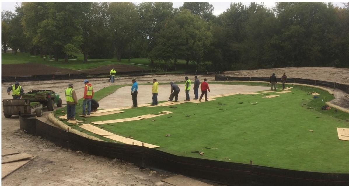
*Figure 2. Erosion and sediment control during construction helps to protect water quality from runoff during construction at Oak Hills Country Club. Photo Credit: Dan Maddox.*
