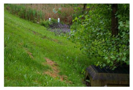
Figure 4. Grassed filter strip to infiltration basin.
