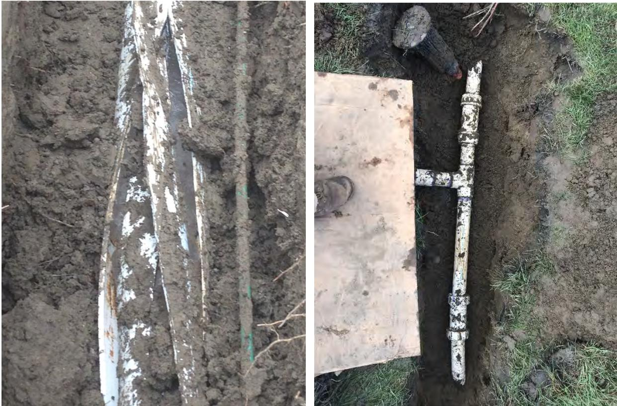
*Figure 8. Irrigation system break (left) and repair (right).*
