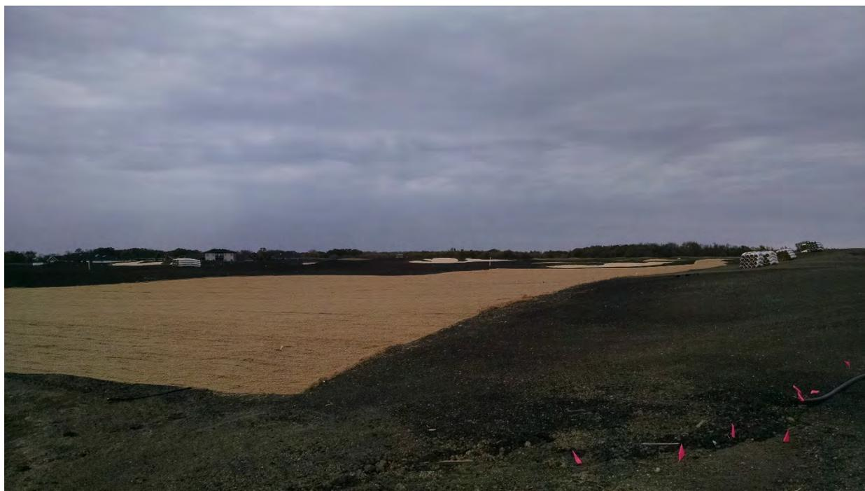
*Figure 3. Erosion mat.*
