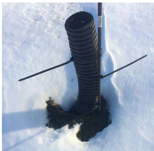
*Figure 9. Keeping drain basins open throughout the winter allows melt water to infiltrate and flow properly during spring melt.*
