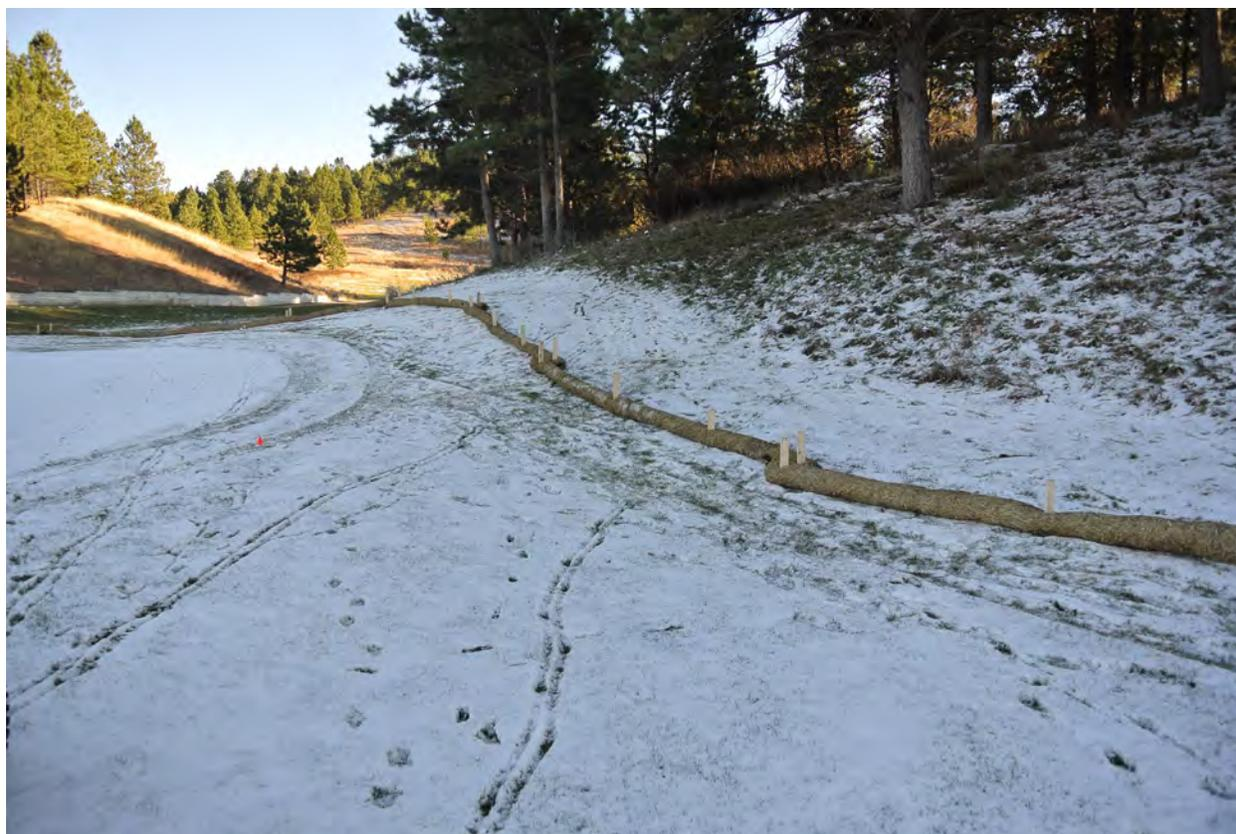
*Figure 1. Erosion control during construction is a regulatory requirement.*
