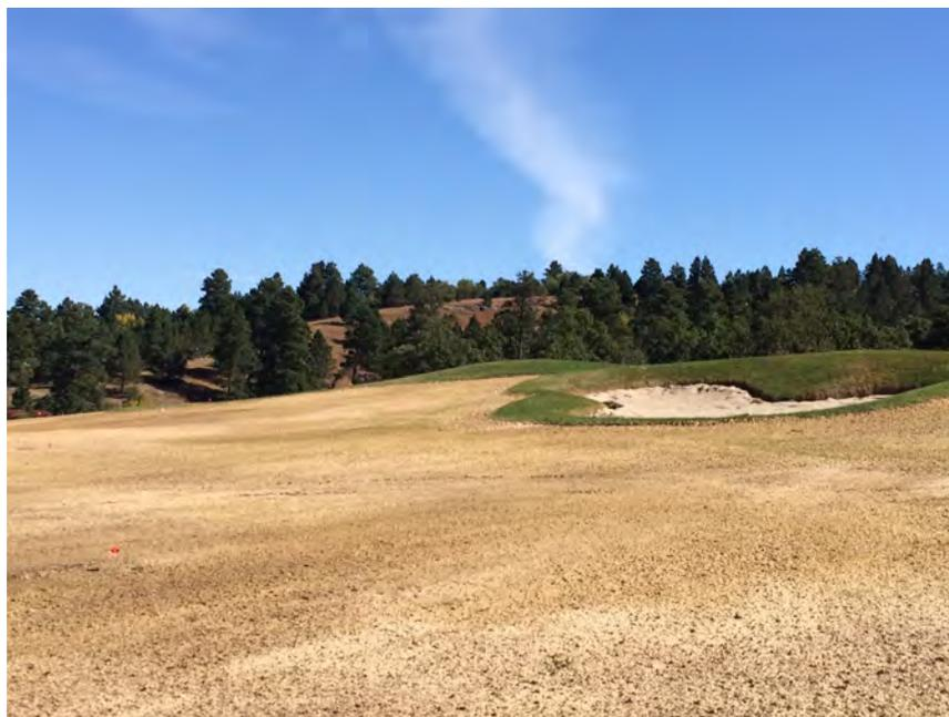
*Figure 11. Hydromulch cover on a sloped site reduces the potential for erosion.*
