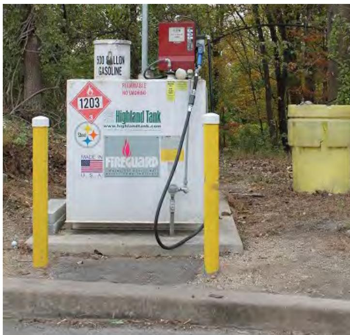
*Figure 35. Fueling station with an AST for fuel storage.*
