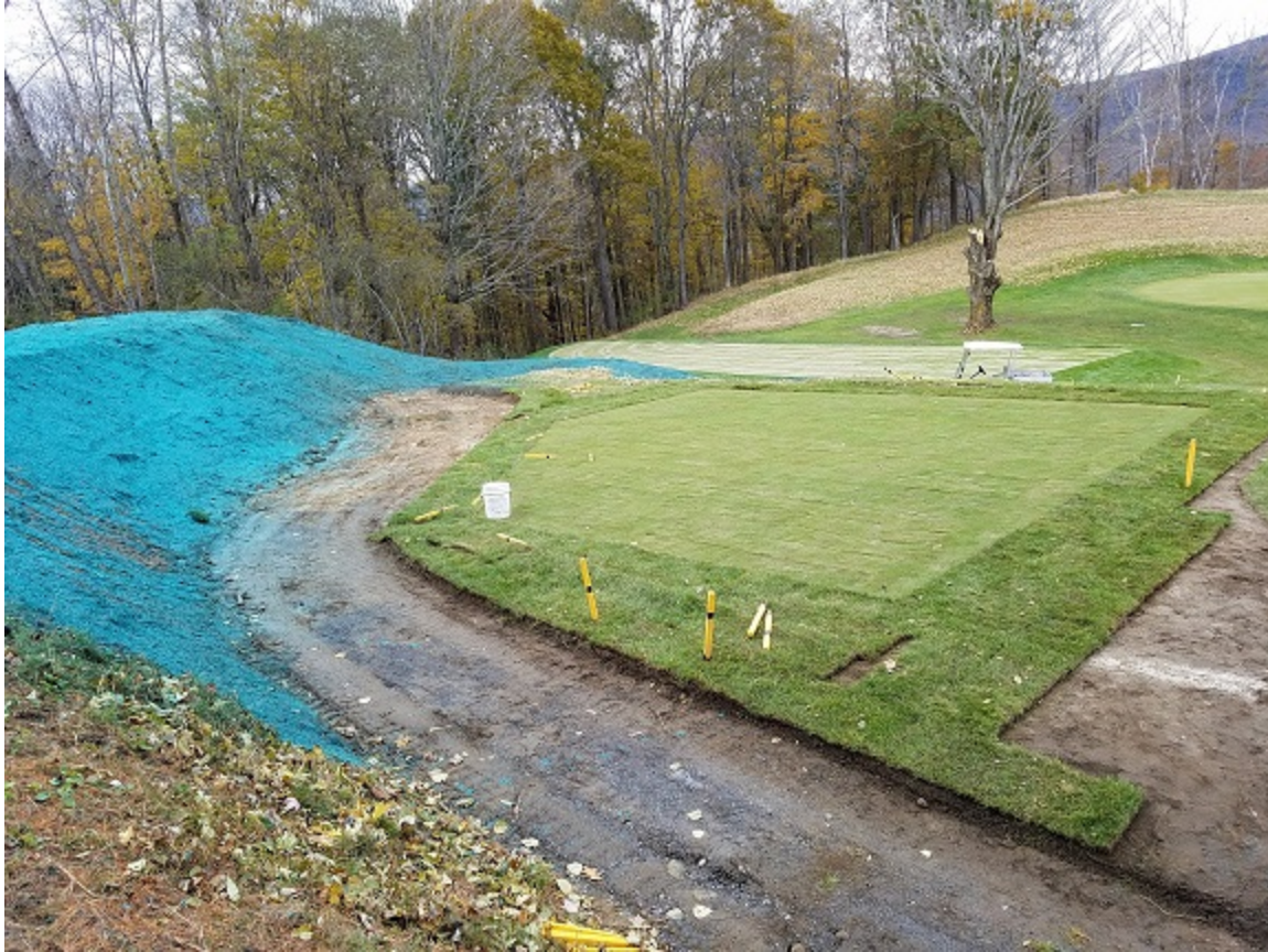
Figure 1-2. The tee was sodded, while the tee surround was hydro seeded to help prevent erosion and stabilize the soil, during the winter months.
