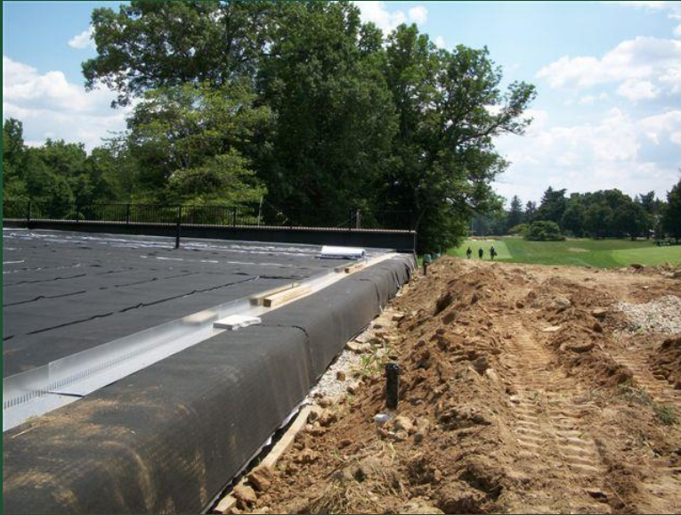
Drainage fabric on the roof
