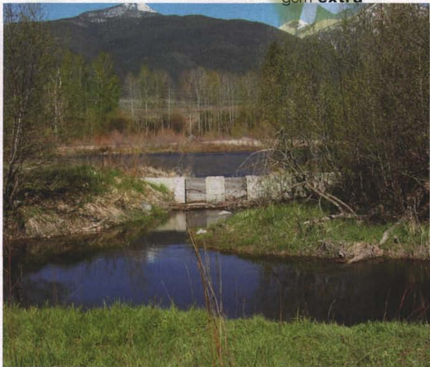
Above left: Michael Brandon, Class A superintendent at White Tail Golf Course. Above: A weir that divides the Bitterroot River and Middle Burnt Fork Creek. The weir is no longer functional and water spills over it during severe floods.
